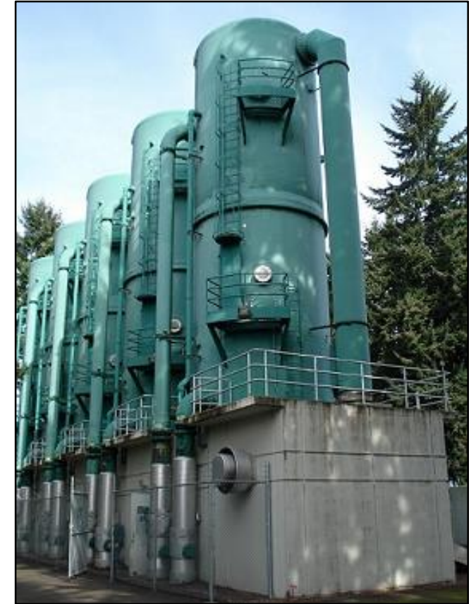
Groundwater treatment aeration towers, Vancouver Waster Station 1 Superfund Site, WA.
