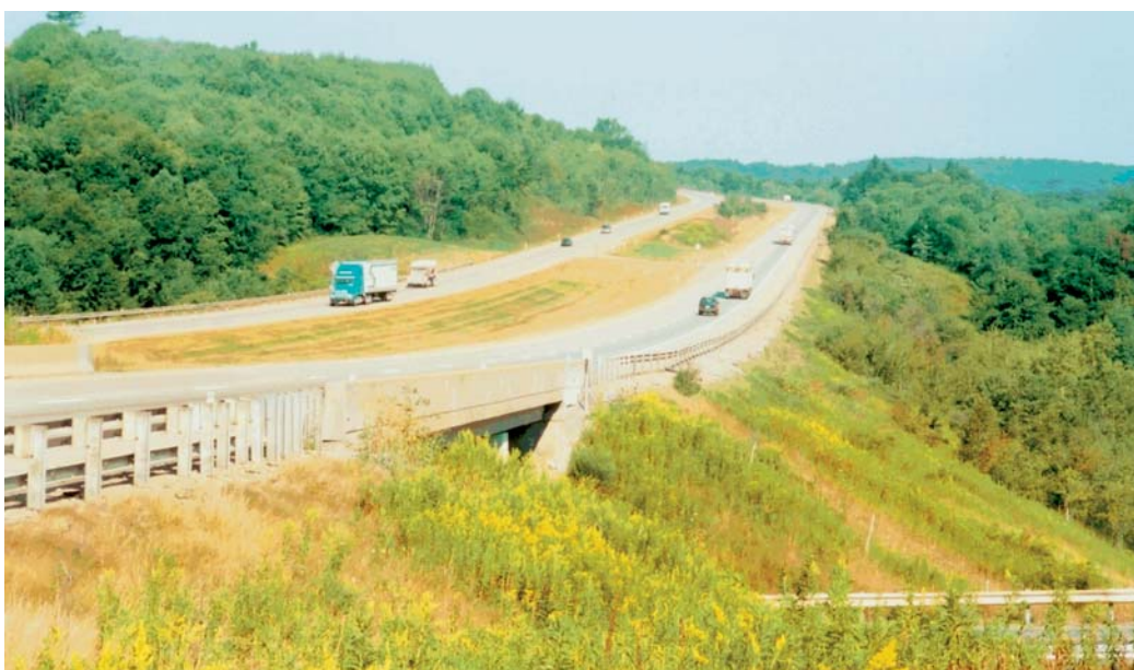
I-80 west-bound over SR 0338 looking West
