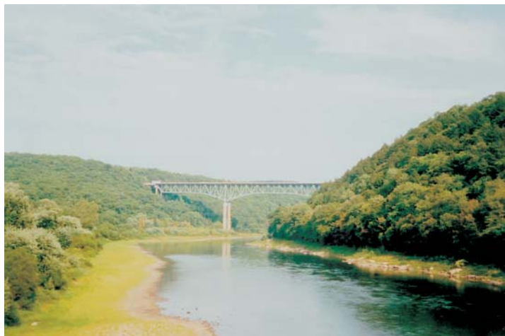
I-80 over Allegheny River looking South
