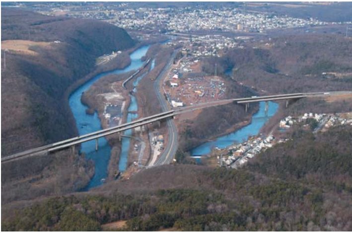
Lehigh and Pohopoco River Bridges
