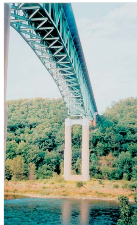
I-80 over Allegheny River looking North
