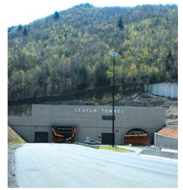
Lehigh County Tunnel
