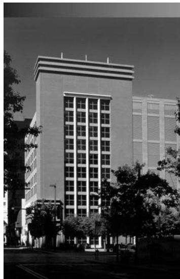
Project Highlight: Theater Square Parking Garage Mascaro's use of the design-build delivery method to change the structural system from precast concrete to post-tensioned, cast-in-place concrete was key to this project's success.
