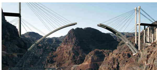
Fig. 5 - Stayed Arch Erection
