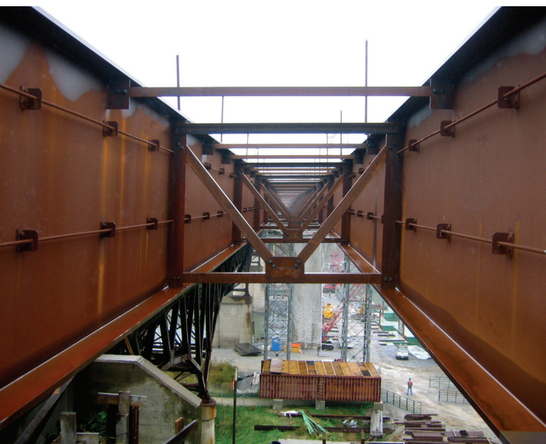
Figure 3. Correct diaphragm configuration for deep girders as utilized on the new James Rumsey Bridge.
