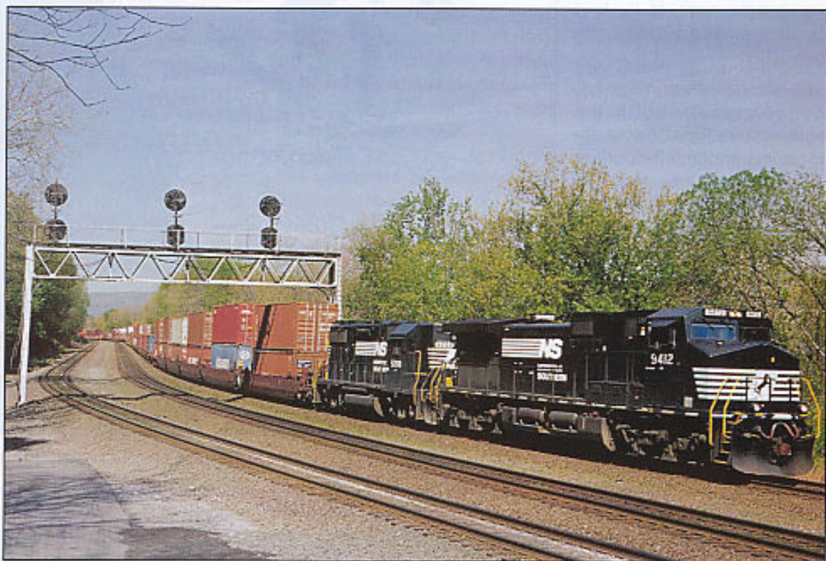
Eastbound Doublestack Approaching Rockville Bridge
