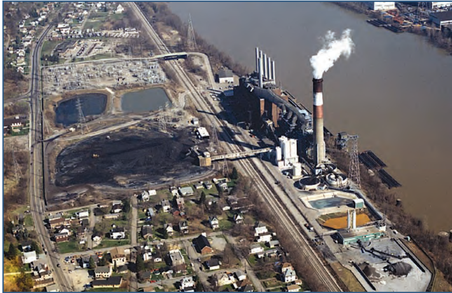
Phillips Power Station along the Ohio River across from Leetsdale, PA was the site of the first Flue Gas Desulfurization Scrubber on a Utility Power Plant in the U.S. The plant was owned at that time by Duquesne Light. The white plume from the stack is water vapor from the wet scrubber process. (Photo courtesy Reliant Energy)
