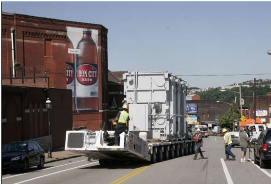
Moving the massive new 350 MVA transformer up Liberty Avenue into the company's Arsenal substation.
