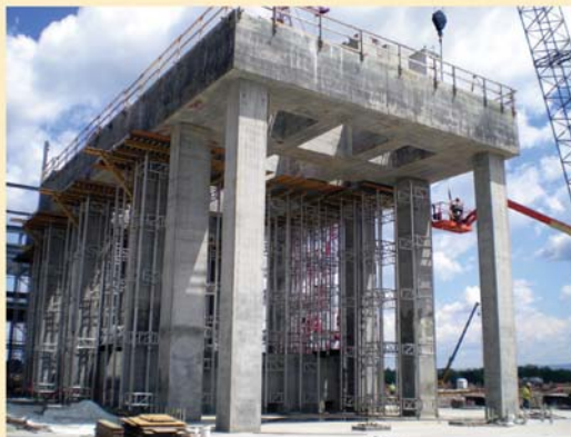
Turbine Pedestal Foundation
