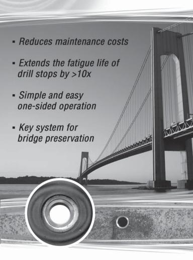
FTI's StopCrackEX system cold expands a bushing into a drill stop, imparting residual compressive stresses around the hole - which protects it from cyclic loads and arrests further crack growth.
