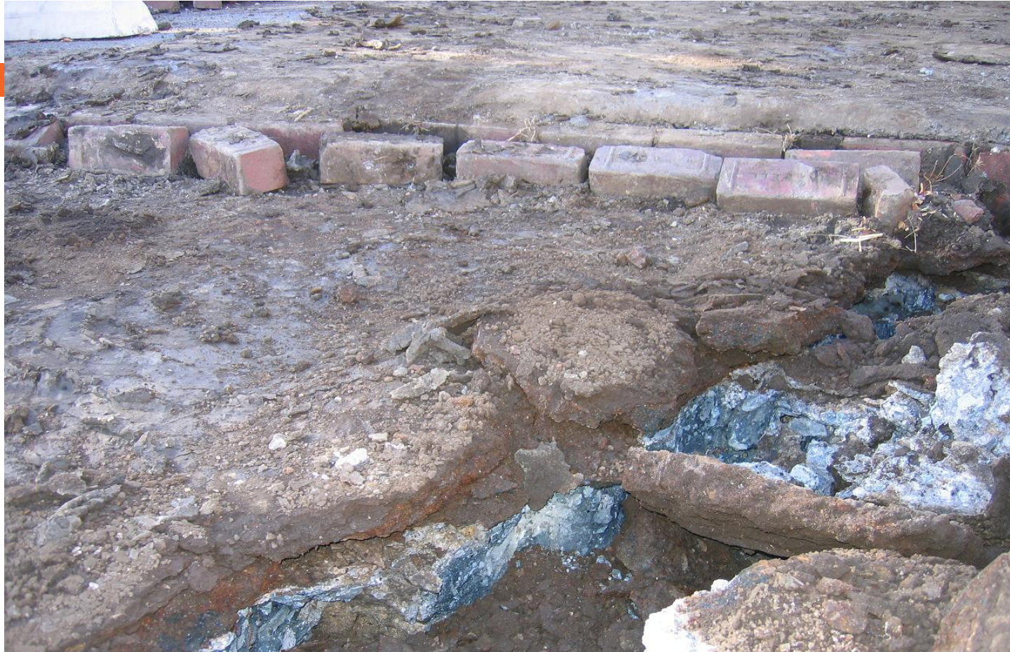
Demolition layers: 3" asphalt, 3" brick, 4" fly ash, 8" concrete
