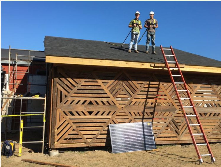
Coalfield Development Corporation Solar installation demonstration. Huntington, WV
