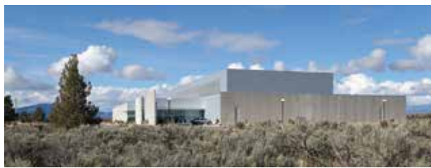
Exterior view of Facebook's Prineville, OR Data Center
