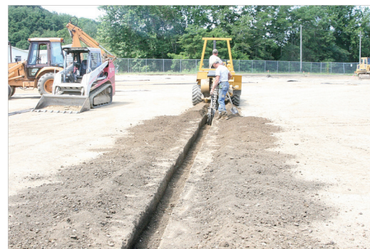
Turf trenching for natural grass field underdrains
