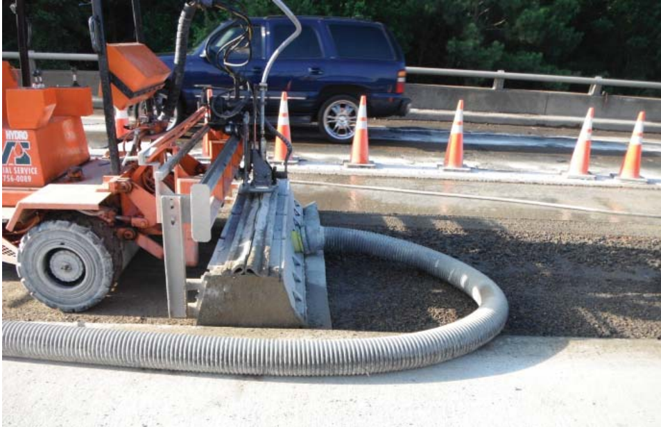
Hydromilling in Preparation for Placement of Overlay
