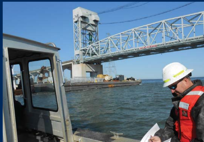
James River Bridge – Newport News, VA Inspection, Evaluation and Rehabilitation
