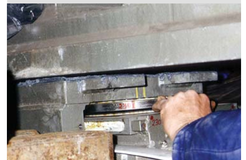
Large gaps between steel structures are compensated with MM1018.
