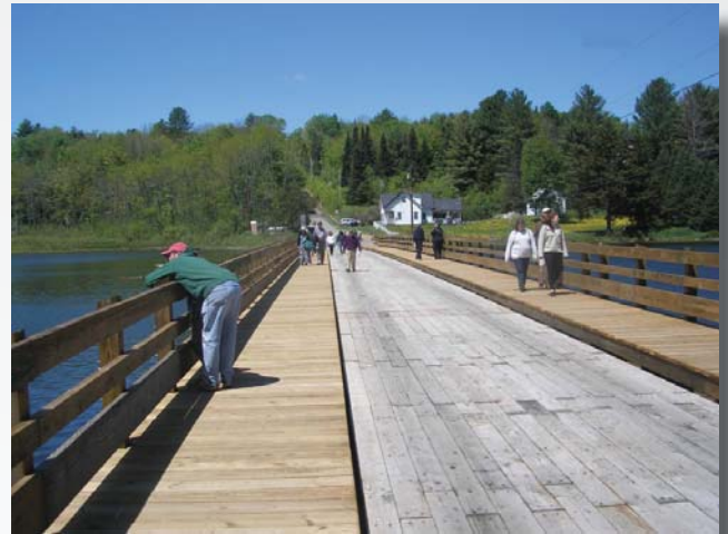
Brookfield Floating Bridge
