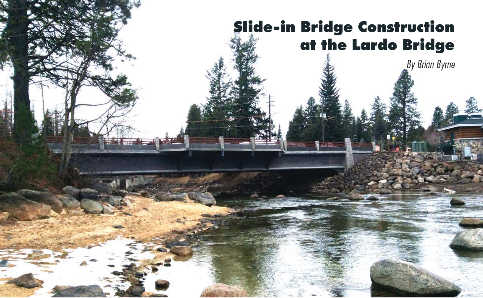
Northern Elevation of Completed Lardo Bridge
