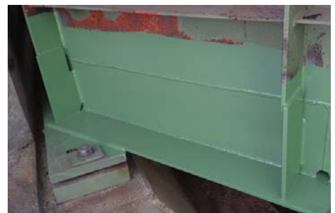
Steel Girder after Repair
