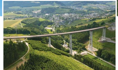
Nuttlar Viaduct on Germany's A46 motorway, was built using MM1018 resin.
