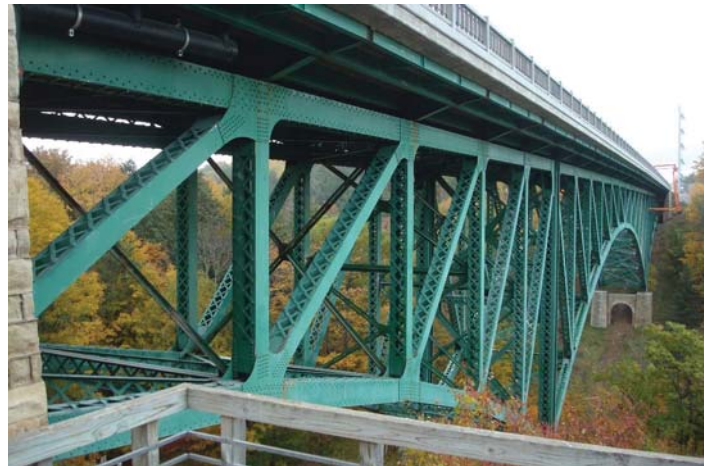
Cut River Bridge Elevation
