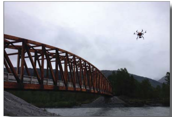
Drone in Action over the Placer River Trail Bridge (Photo courtesy of the USDA Forest Service)
