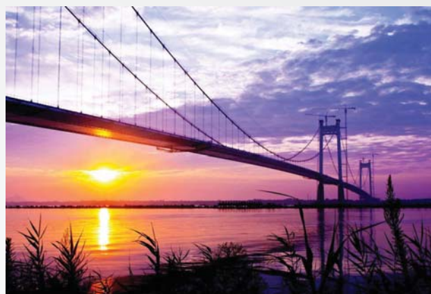
Ma-an-shan Yangtze River Bridge
