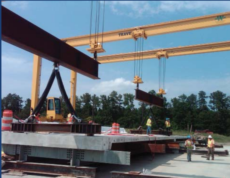
PCU Erection
