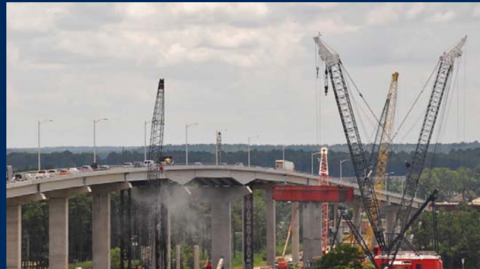
Dominion Boulevard – Chesapeake, VA Construction Engineering and Inspection
