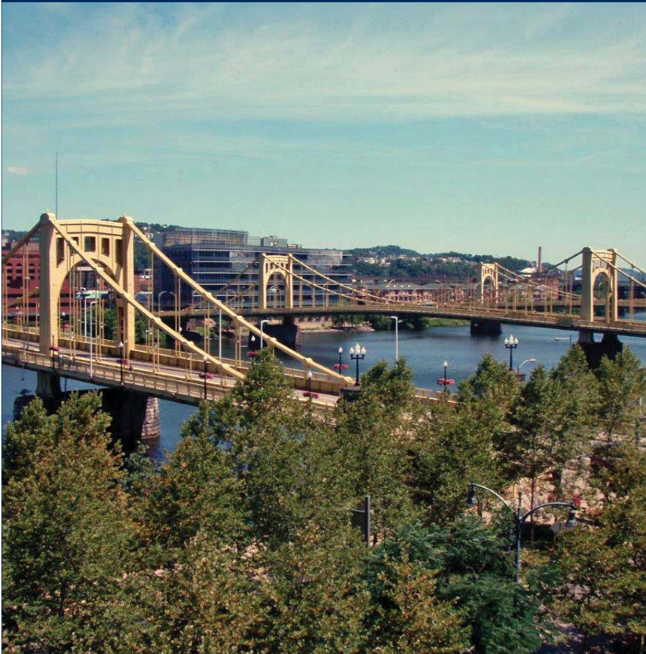
6th, 7th and 9th St. Bridges – Pittsburgh, PA Inspection, Analysis and Rehabilitation
