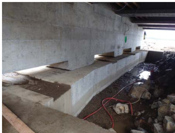
Abutment on Slide Slab after Bridge Move
