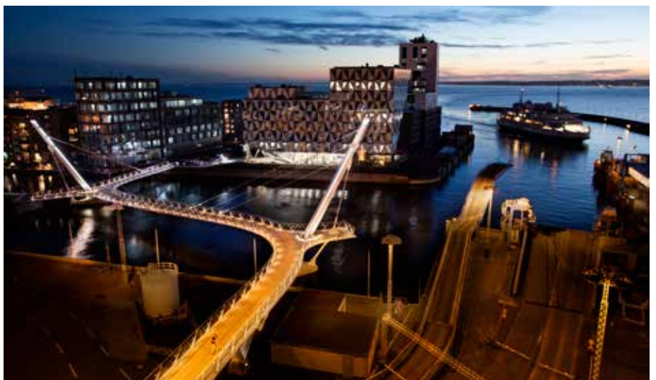
Varvsbron (the shipyard bridge); Helsingborg, Sweden
