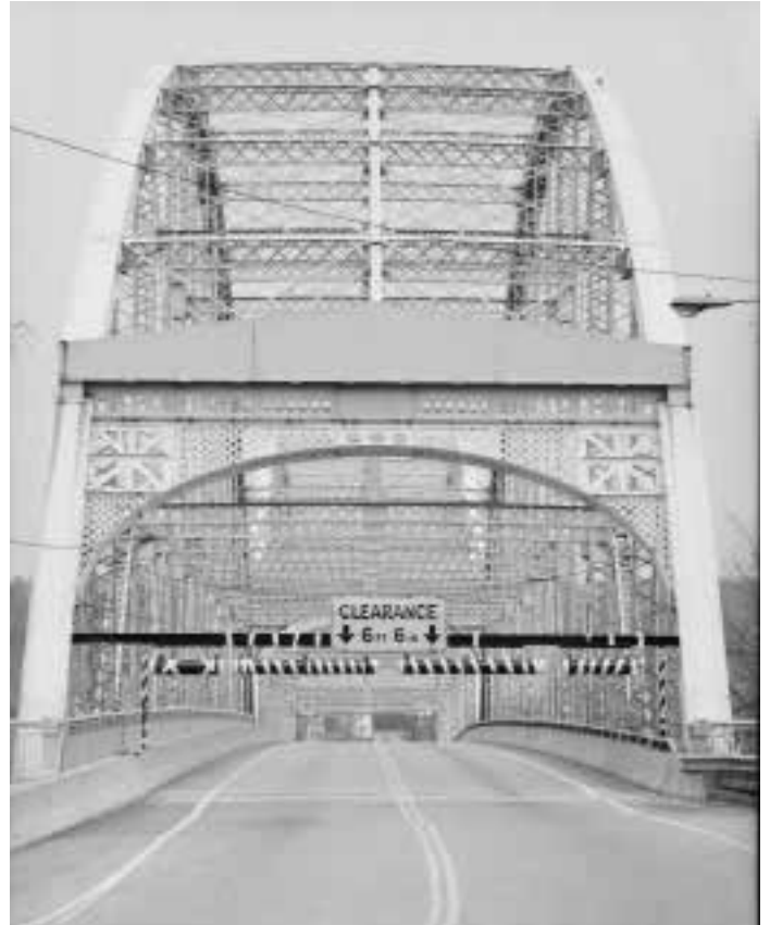
6th Street Bridge over Allegheny River, Pittsburgh, PA (1892) by Theodore Cooper; later (1927) transported downstream to new location on the back channel of Ohio River at Coraopolis, PA
