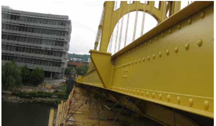
Rachel Carson (Ninth Street) Bridge Rehabilitation; Pittsburgh, PA, USA
