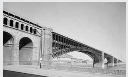
Eads Bridge spanning the Mississippi River, St. Louis, MO (photo courtesy of the Library of Congress)
