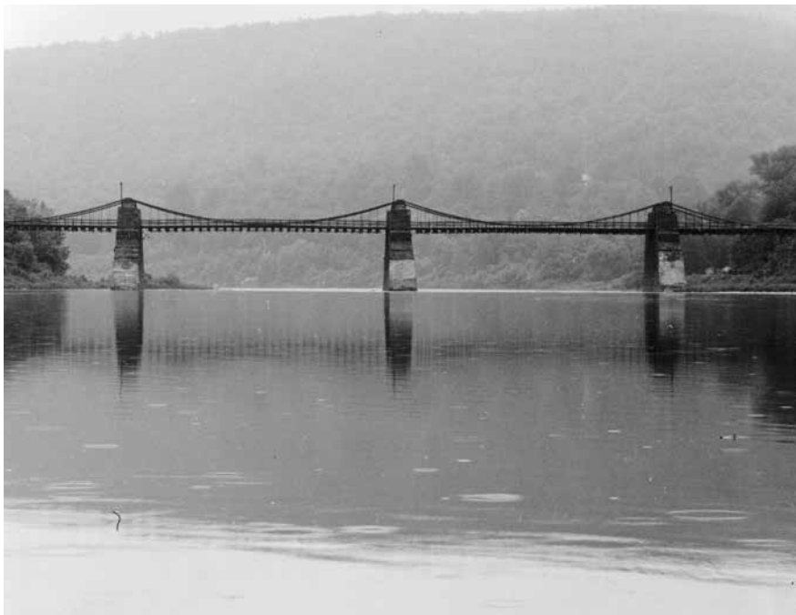
Delaware Aqueduct (1848), Spanning Delaware River, Lackawaxen, Pike County, PA; design is similar to the 1845 Monongahela River Bridge and other early Roebling Bridges; Photo Courtesy the Library of Congress
