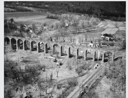
Starucca Viaduct, 1848, Susquehanna County, PA (photo courtesy of the Library of Congress)
