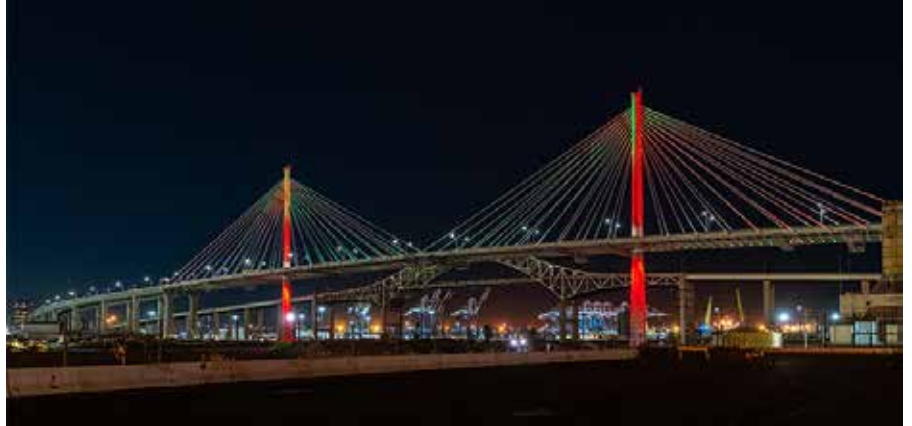
Gerald Desmond Bridge Replacement; Long Beach, California, USA
