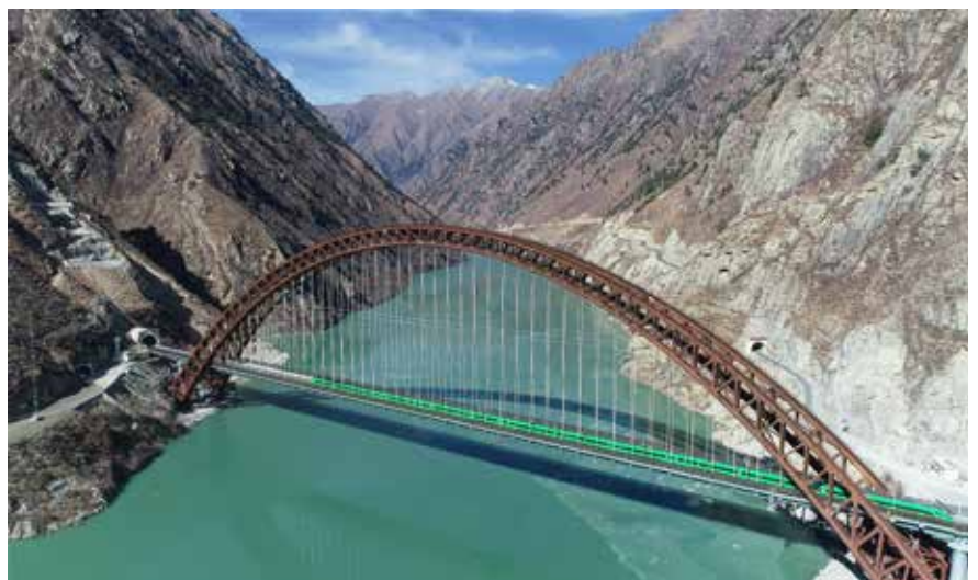
Zangmu Yarlung Zangbo River Bridge; Jiacha County, Shannan City, Tibet, People's Republic of China
