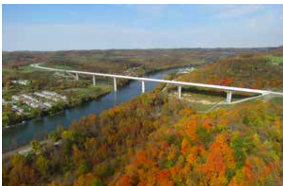
Photo Courtesy of Gannett Fleming, Inc.
