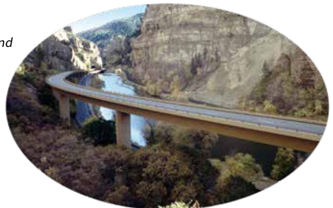
Hanging Lake Viaduct carrying I-70 along the Colorado River through an extremely steep and narrow portion of Glenwood Canyon. EB: 1,308', WB 7,121'
