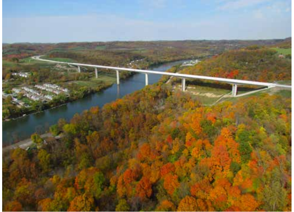
PA Turnpike, Toll 43 over the Monongahela River in Brownsville, Pennsylvania (completed in 2012) is a cast in place, balanced cantilever, post-tensioned, segmental, major river crossing in western Pennsylvania.
