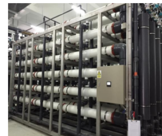
18 Modules per Train x 16 Trains System Installation (1 of 16 Trains Shown)
