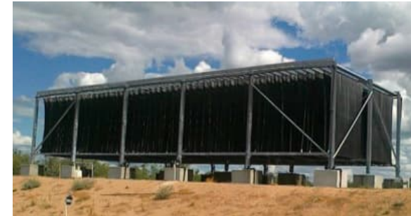
Wind aided intensified evaporation (WAIV)
