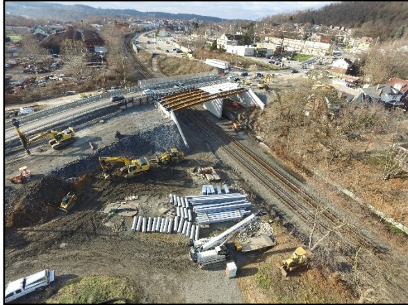
Utilization of Temporary Bridge During Construction
