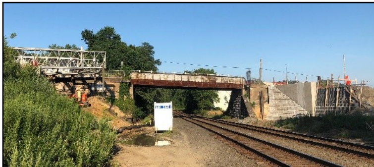
Use of Wing Walls as Temporary Abutments
