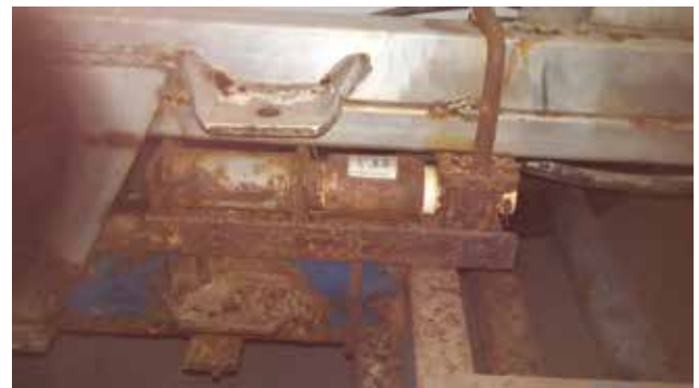
Figure 6: Corrosion on an after-market weigh cell on a fertilizer spreader after 1 year of service
