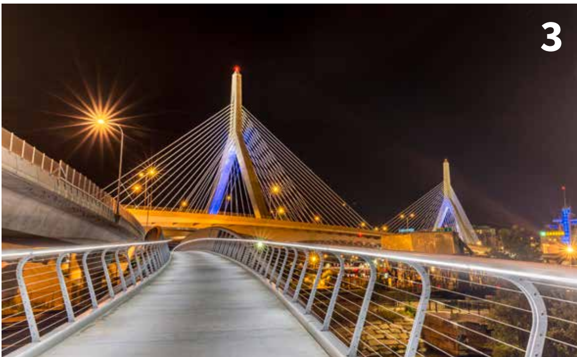
3. North Bank Bridge; The North Bank Bridge is a pedestrian walkway under the cable stayed Zakim Bridge in Boston. Spanning 690 feet, it crosses the MBTA rail tracks; Submitted by: Damian Silverstrim
