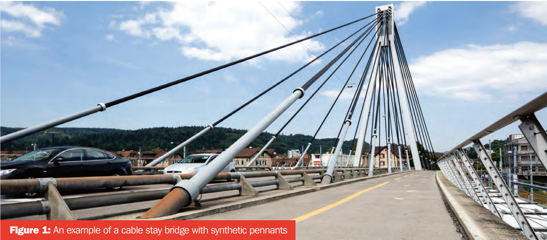
Figure 1: An example of a cable stay bridge with synthetic pennants
