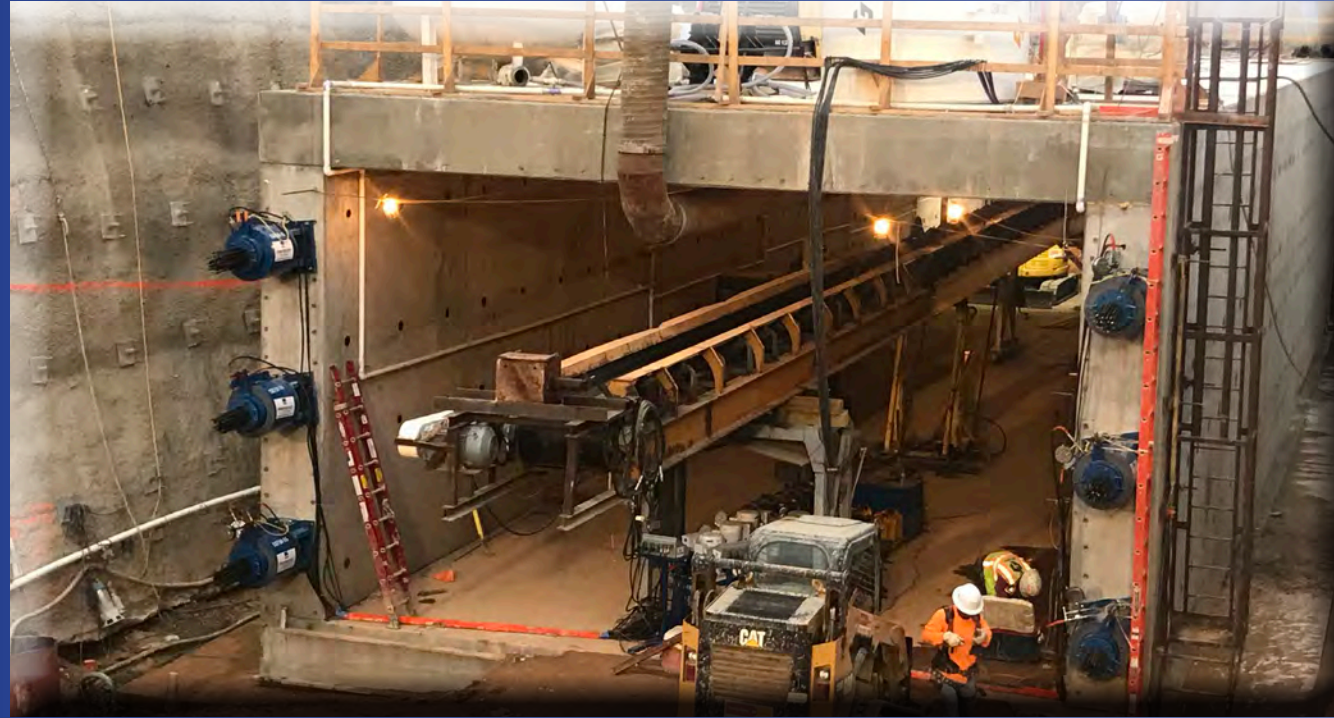
Tunnel Jacking under Live Traffic, GA 2019
