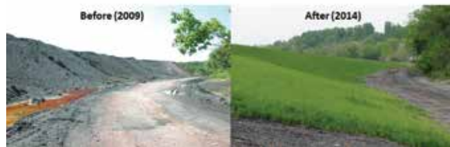
Bauxite residue for acidic coal refuse pile reclamation demonstration at Mather Mine (PA)
