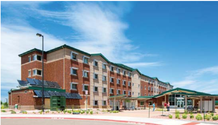
Building south facade with hot water solar panels atop the mechanical room
