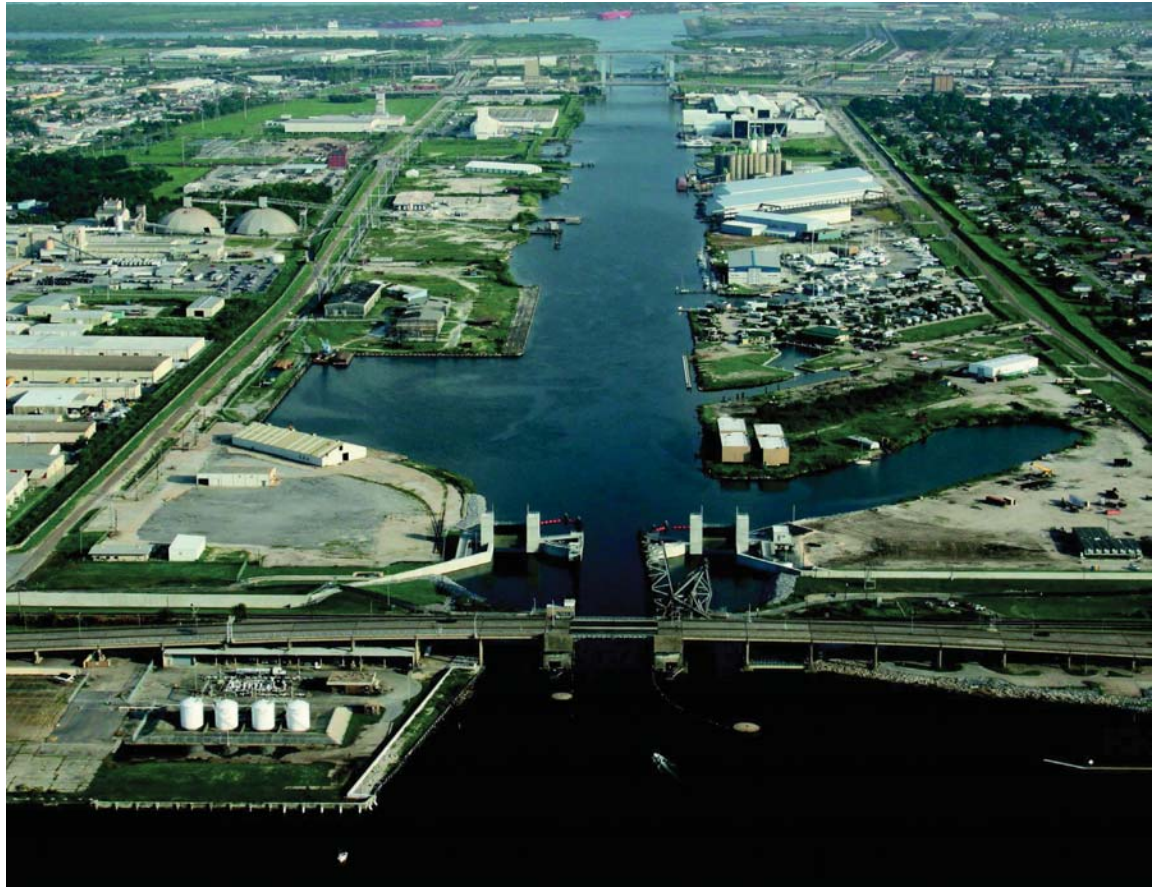
The Greater New Orleans Hurricane and Storm Damage Risk Reduction System built after Hurricane Katrina was tested during Hurricane Isaac in 2012, proving able to mitigate intense storm surge and rainfall. Now, the focus in the delta is shifting from repair and recovery to a broader framework that addresses how to manage the coast and city in a rapidly changing landscape.
