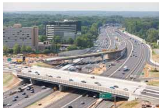
I-495 and Route 7 in Tysons Corner
