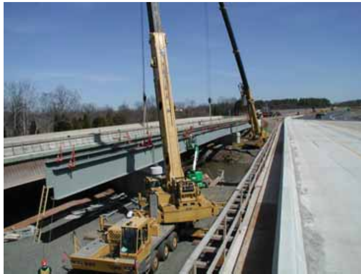
Dulles Greenway Under Construction
