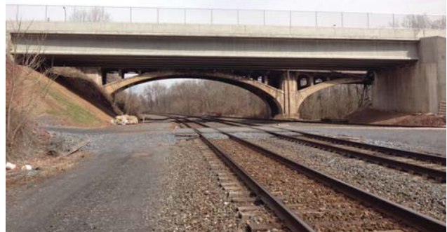
New Birdsboro Bridge over Norfolk Southern Railroad
