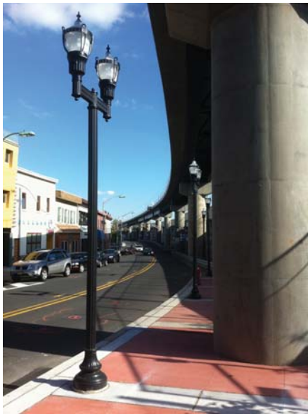
Northern section of viaduct as seen from Avenue E, facing North.
