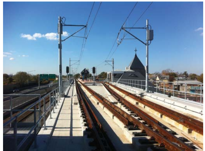
Viaduct turnout section in the approach to the loading platform, facing South.
