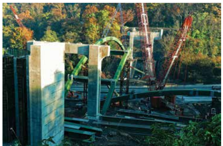
Erection of Structural Steel for New Arch over Weekend in November 2016
