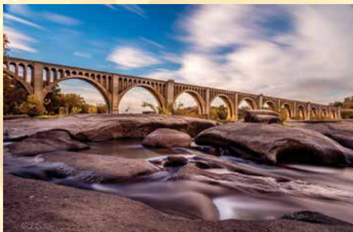
2 nd Place: CSX A-Line Bridge over the James River, Richmond, VA Photographer: Damian Silverstrim "Fantastic contrast ... Great composition ... Surreal reality"
