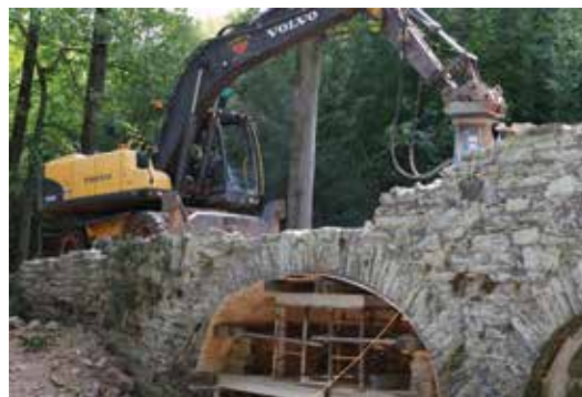
Removal of failed third span arch
