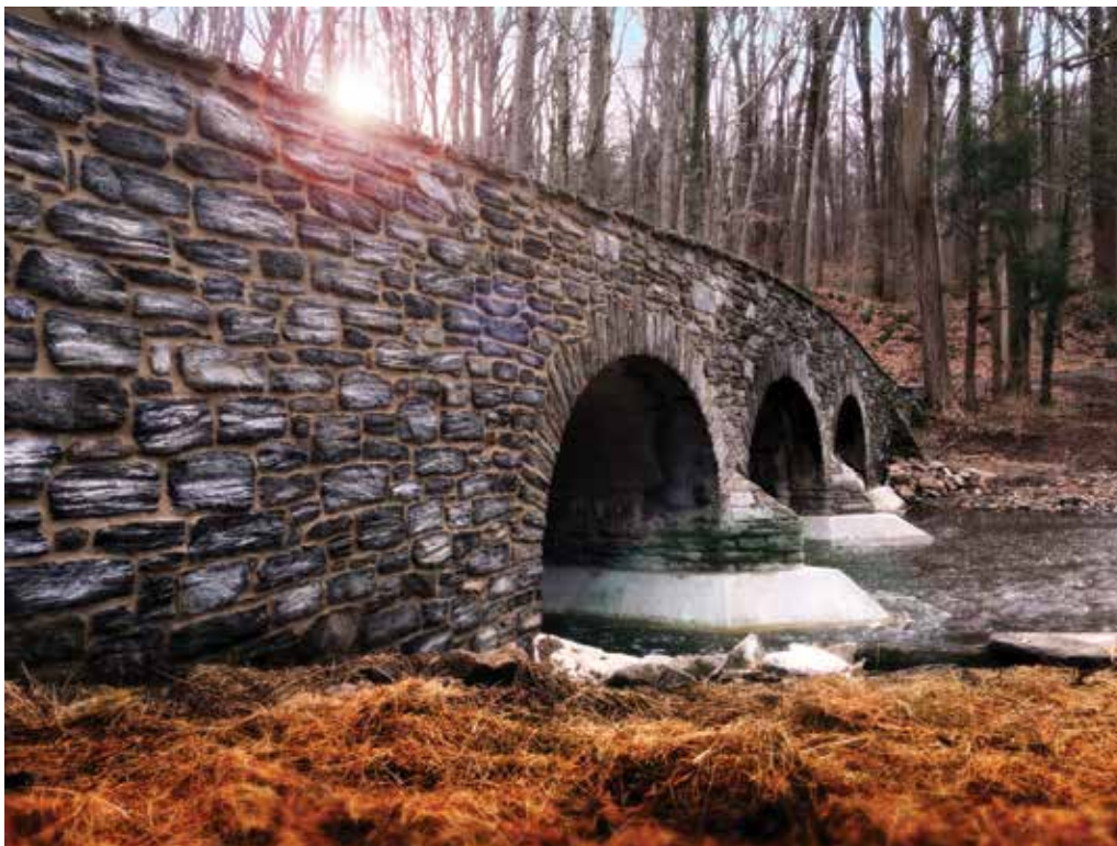
Furness Bridge After Rehabilitation
