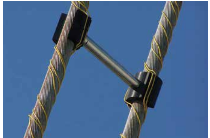
Hanger Separator between the Two Strands
