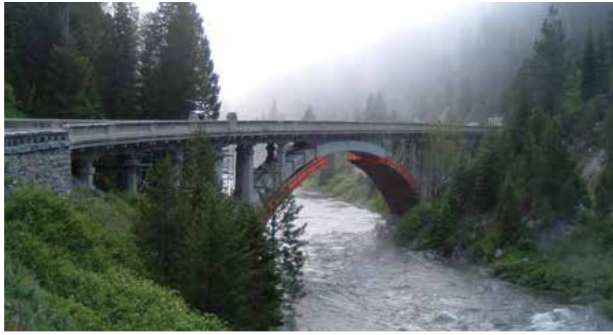
Chloride Extraction – ECE Process – During Construction
