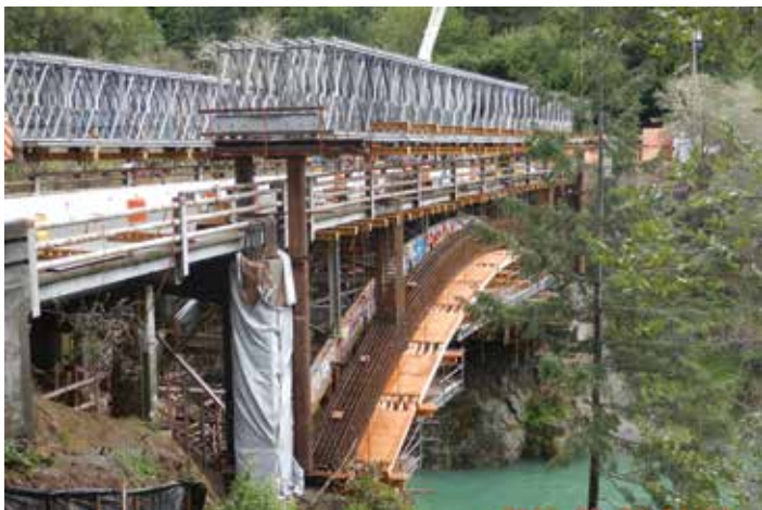
Looking upstream during one of the arch rib concrete pours as truss bridges support the formwork, reinforcing steel and concrete ribs. Work platforms are hung from the old bridge.
