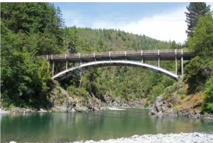
The original bridge viewed from downstream.
