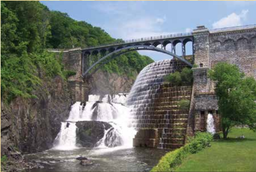
4 th Place: Croton Reservoir Dam Bridge over the Croton River, Croton Gorge Park, Croton-on-Hudson, NY Photographer: Richard Cochrane "Wonderful capture of light ... you can almost hear the roaring Croton River"
