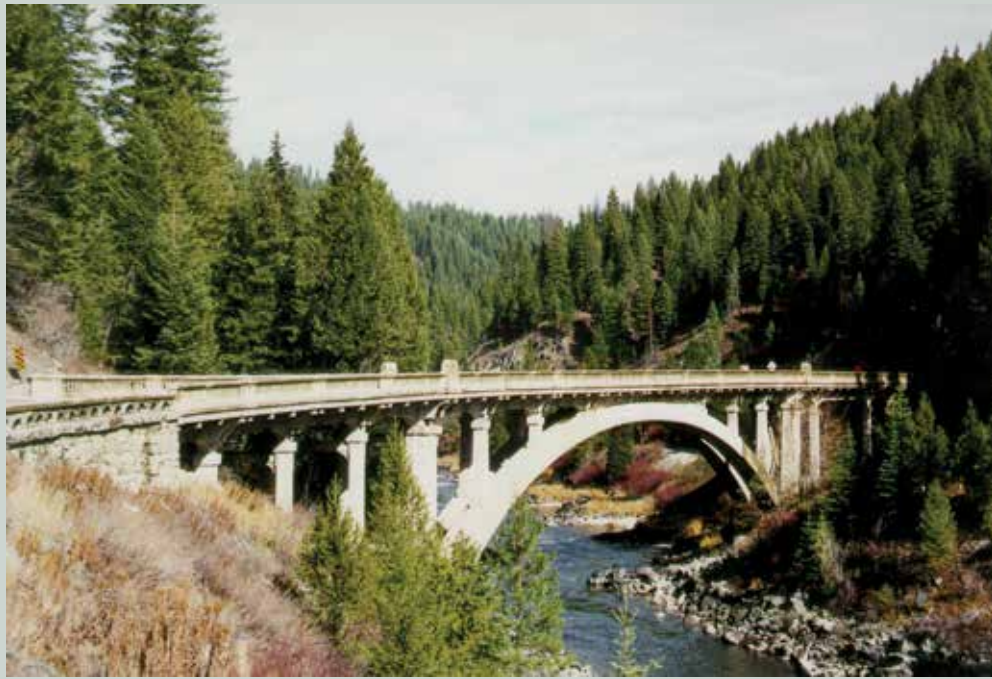
The Historic Rainbow Bridge over the Payette River — after mitigation
