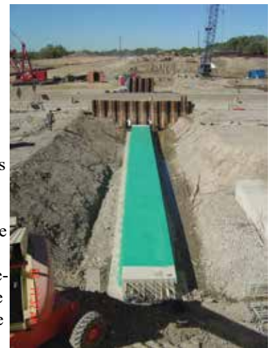
Exterior Longitudinal Foundation Tie with Waterproofing Coating
