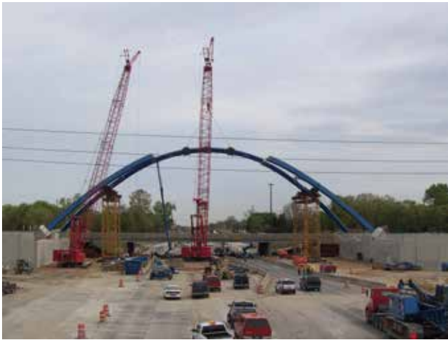
Erection of the Middle Segment of the Arch Rib
