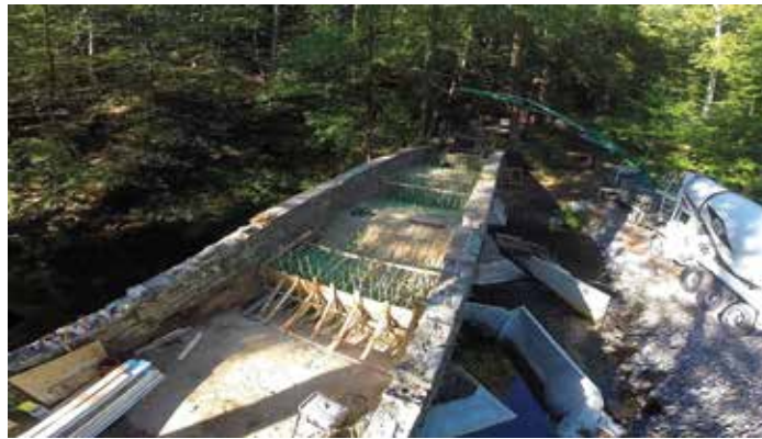
Fill removed over Spans 1 & 2
