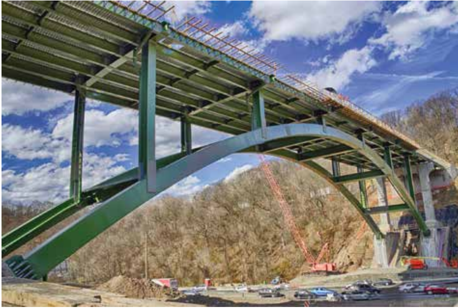
Structure After Completion of Steel Erection
