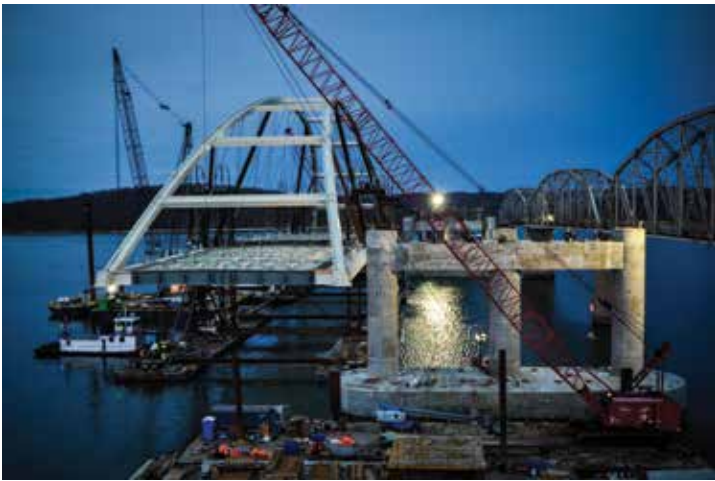
Kentucky Lake Arch Lift
