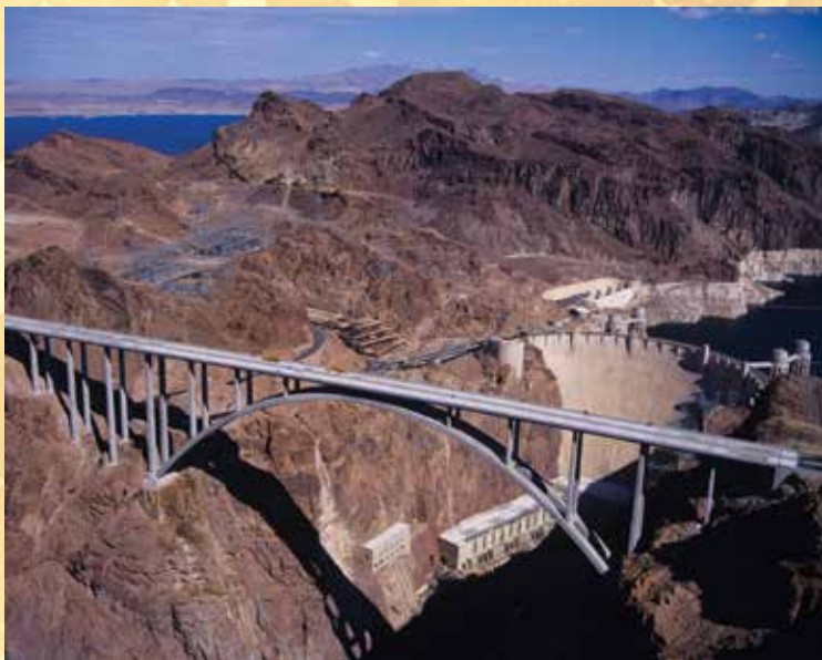
7 th Place: Mike O'Callaghan-Pat Tillman Memorial Bridge over the Colorado River, Arizona/Nevada Border Photographer: US Bureau of Reclamation for Federal Highway Administration "Lots of drama ... Excellent composition"
