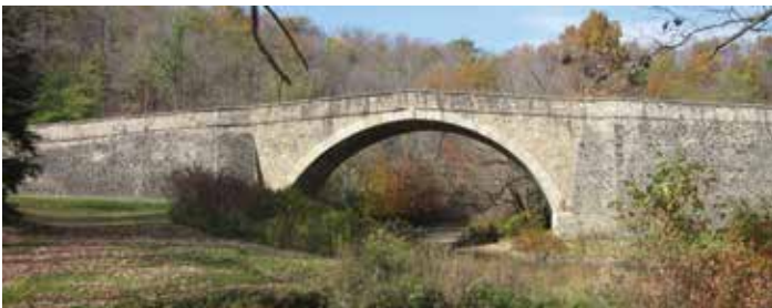
Little Crossings Bridge, National Road (US 40) spanning the Casselman River, Casselman State Park, Grantsville, MD. Photo courtesy of the Editors.
