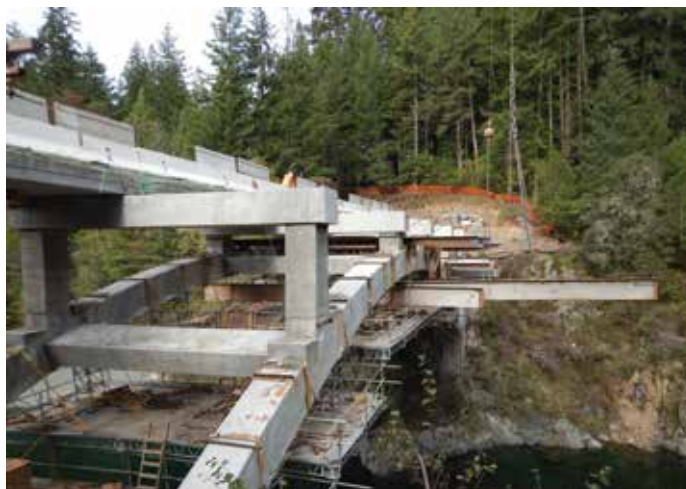
The photo shows the upstream view of the completed arch ribs, columns, cap and struts before the Stage 2 superstructure was constructed. The existing bridge has been demolished and removed.
