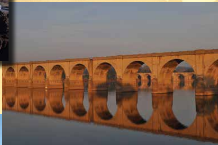
8 th Place: Norfolk Southern RR Bridge over the Susquehanna River, Harrisburg, Pennsylvania Photographer: James Radion "Peacefulness ... Colors and content are striking"
