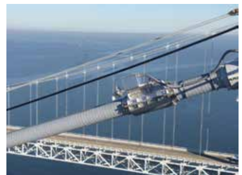
Figure 4 Cable Dehumidification Injection Sleeve location (AECOM)
