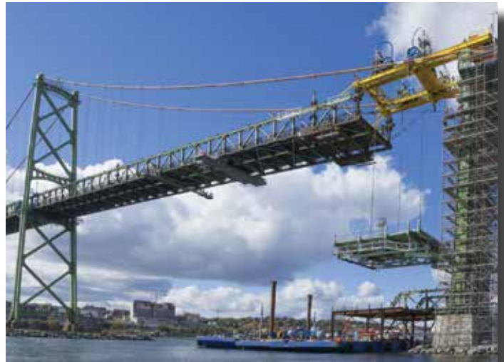
Angus L. Macdonald Bridge
