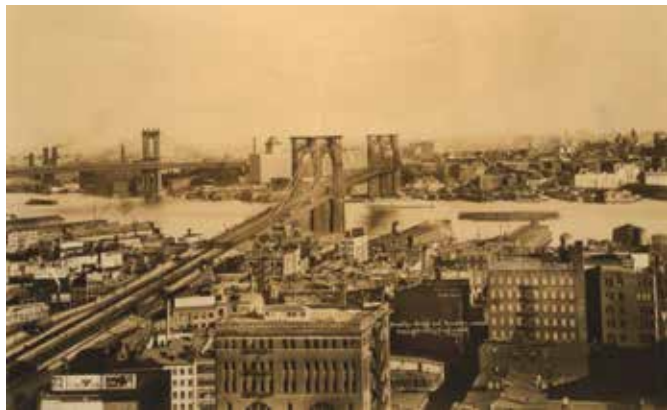
Brooklyn Bridge, c. 1910 Photo Courtesy Library of Congress
