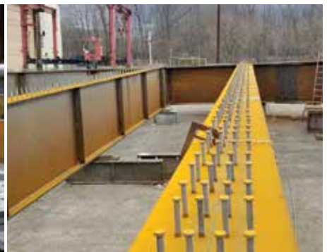
Edge girders and floor beams assembled in the yard
