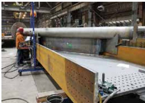
Cable anchor assembly attached to an edge girder in the shop
