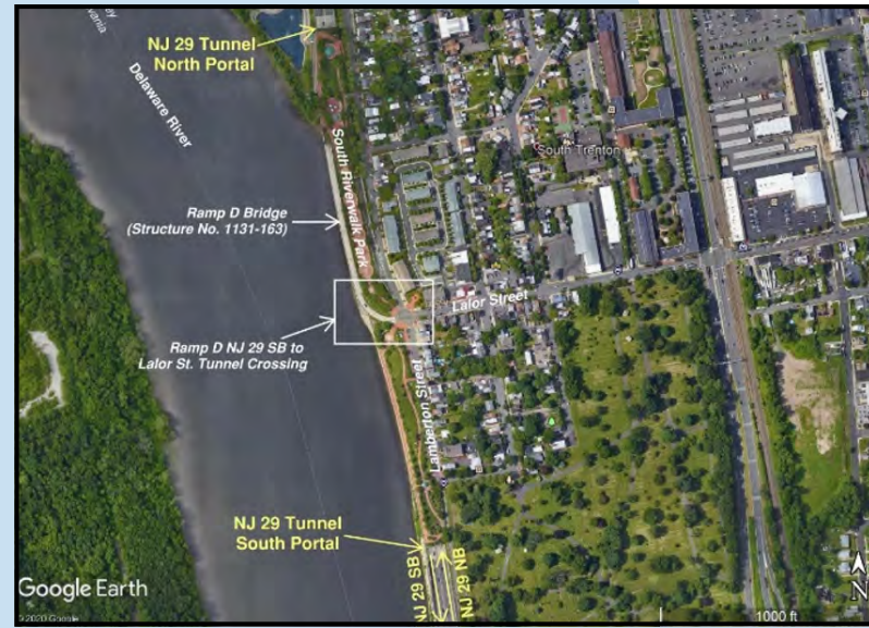
The NJ Route 29 Tunnel is located along John Fitch Way between the Riverview Cemetery and Arm & Hammer Park in Trenton, New Jersey. Access from the Southbound Roadway to Lator Street is provided through the Ramp D Bridge, which crosses over the tunnel and subjects the frame to live load.
