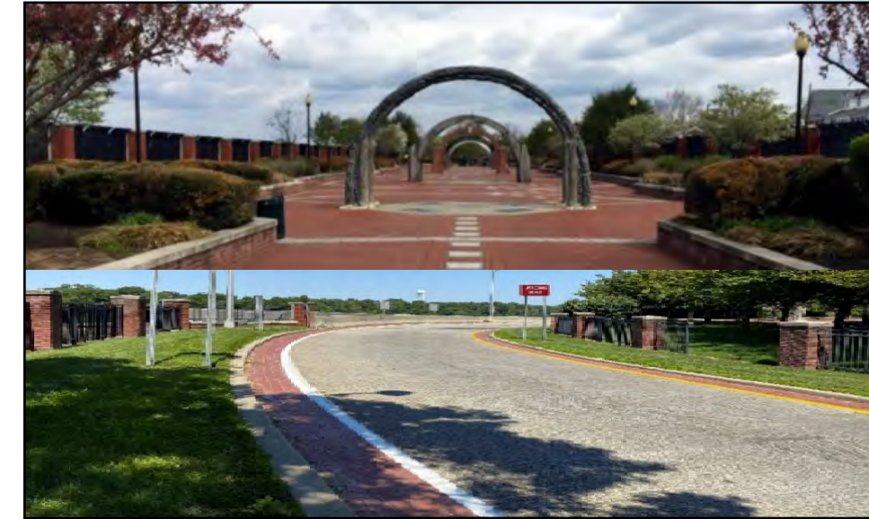
Access to the scenic South Riverwalk Park (top image) is provided by the Ramp D Bridge (bottom image) to the Lambertson Street and Lator Street intersection. Pedestrian and vehicular live loading were considered for the analysis and load rating.
