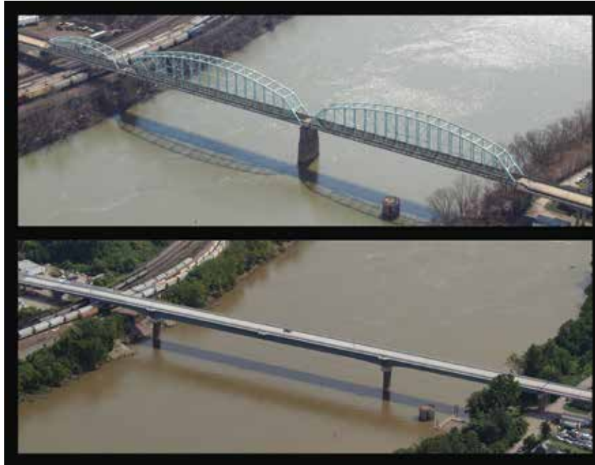
Charleroi Monessen Bridge Before and After
