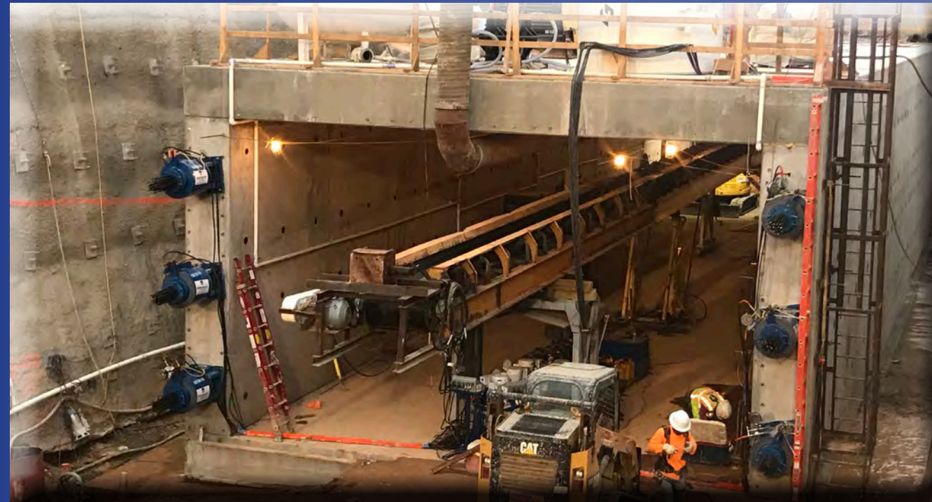
Tunnel Jacking under Live Traffic, GA 2019
