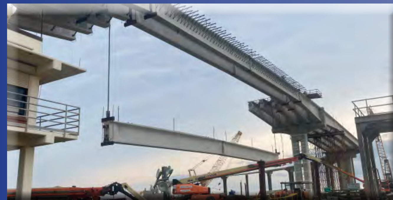
Lifting Precast Beams for the Sargent Bridge, TX 2020
