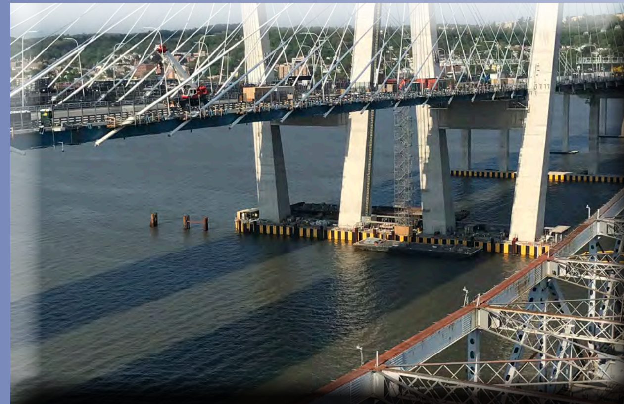
Lowering of the Tappan Zee Suspended Span, NY 2018
